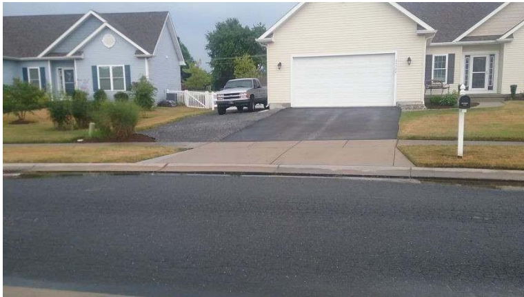
Driveway extension – does not comply – different material
