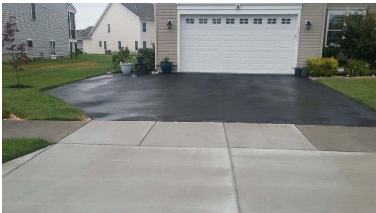
Driveway Extension – Complies same material and location
